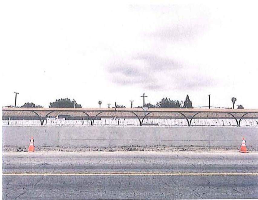
4. Across the street from subject property; facing north at Interstate 5 freeway.
